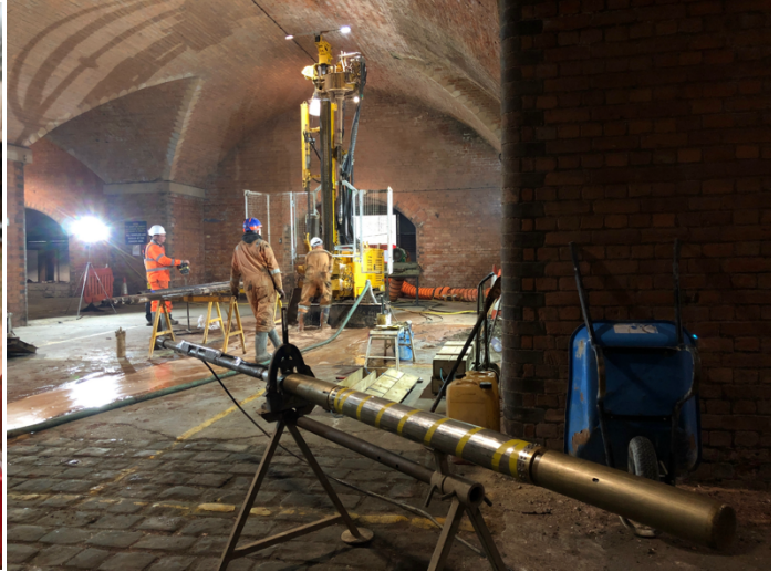
Figure 6. A high pressure dilatometer ready for deployment under a rotary drilling rig. Photo by Cambridge Insitu Ltd, 2022
